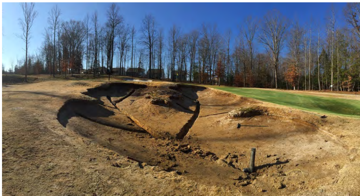
Figure 1. Bunker renovation at Magnolia Green.
