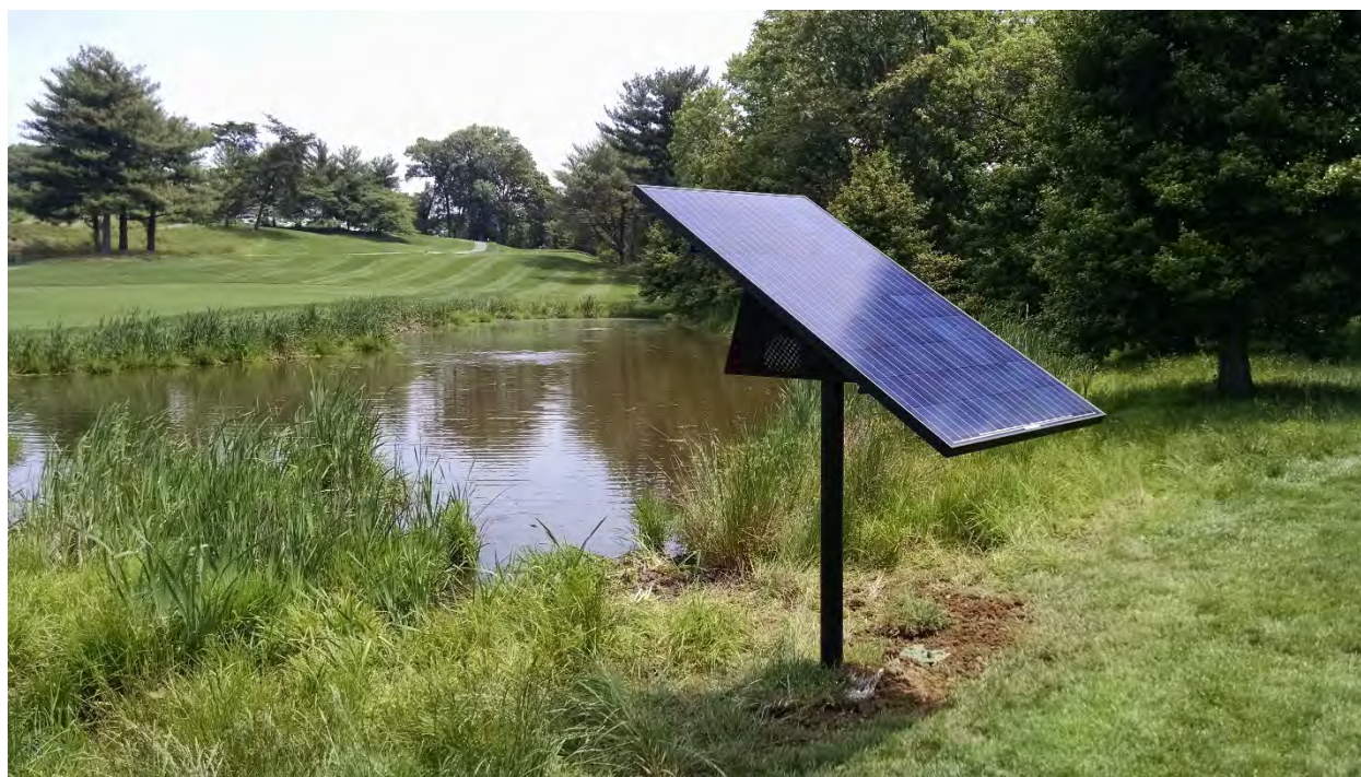
Figure 12. Solar-powered artificial aeration at Army Navy Country Club helps to maintain adequate dissolved oxygen.
