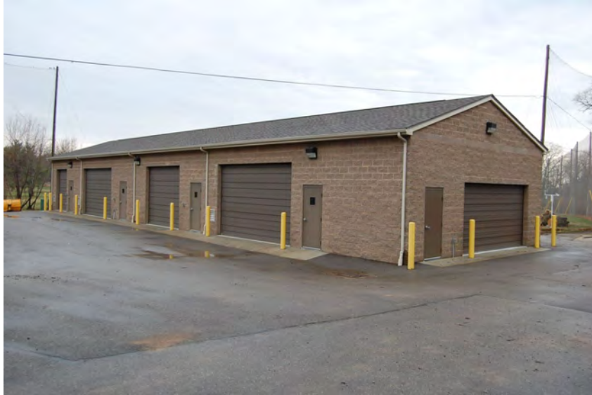
Figure 32. Supply local fire department with blueprint of storage building(s), Material Safety Data Sheets (MSDS) for all product stored in building(s). Photo credit: Jason Mahl.
