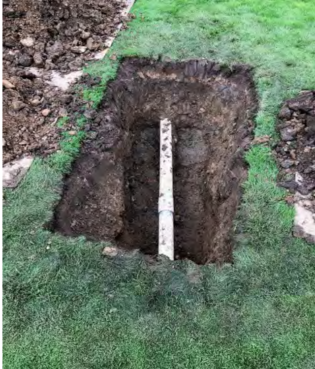
Figure 9. A visual inspection should be carried out for leaks, misaligned or inoperable heads, and chronic wet or dry spots, so that adjustments can be made or replaced. Photo Credit: Ryan D'Autremont.
