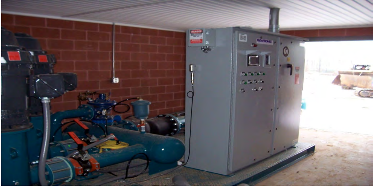
Figure 7. Pumps should be sized to provide adequate flow and pressure. Photo credit: Jason Mahl.
