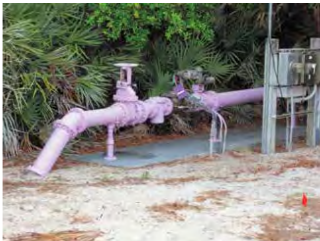
Figure 3-7. Purplish-pink pipe indicating effluent water which is an increasing source of irrigation for many golf facilities.
