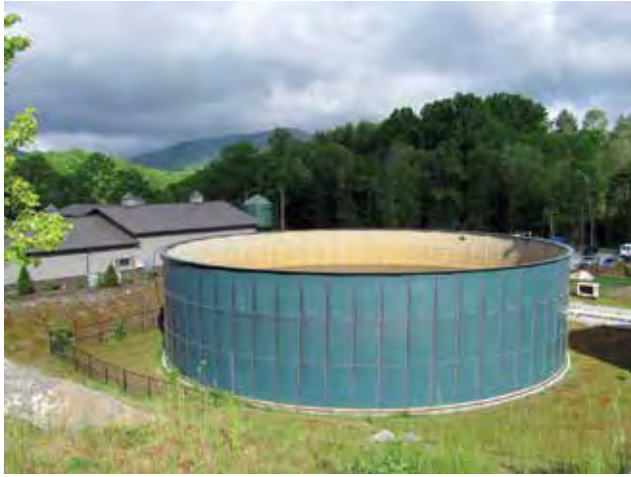
Figure 2-13. Effluent water storage facility on a golf course.
