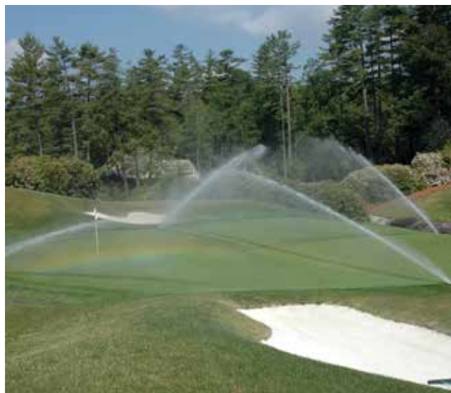
Figure 3-1. A properly designed and operating irrigation system is the life-line for golf facilities. Most are computerized and synchronized with weather stations and/or soil moisture probes to efficiently use irrigation water.
