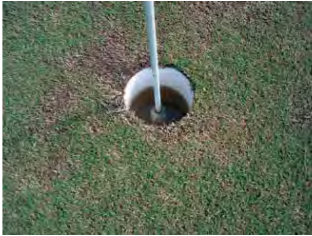
Figure 3-11. Water remaining in a golf pin indicating poor soil drainage.
